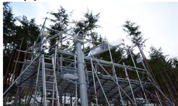
Figure 7. Audio system, Weatherproof digital camera and solar panels placed in Cyber Forest project site.
